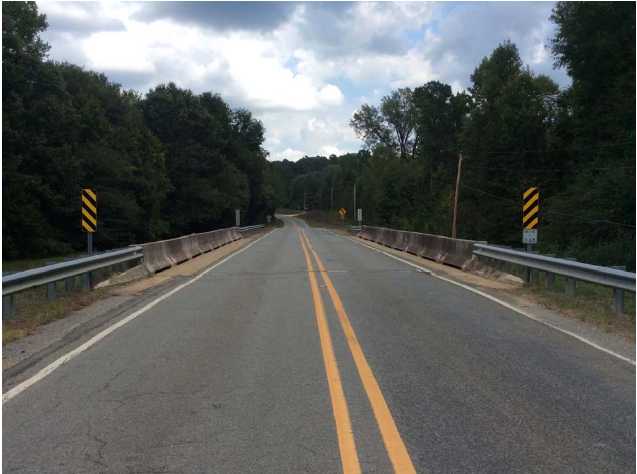
Note: 0.5" ACHM overlay on bridge deck
